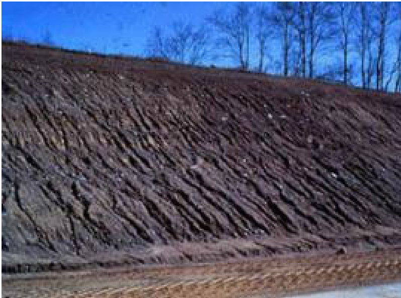
Gully erosion Rill erosion
